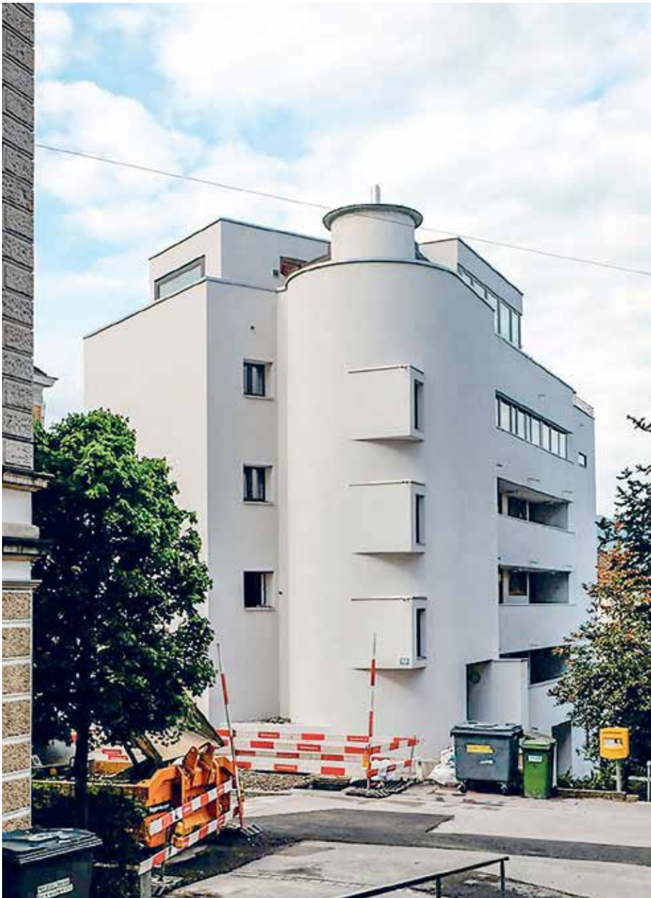
The residential building on Clausiusstrasse in Zurich with its circular stair tower.
