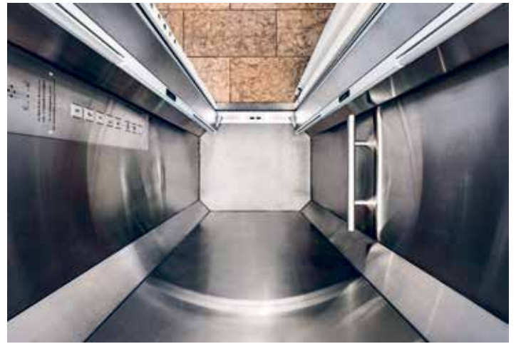
Thanks to the bevelled corners and the folding door, the new cabin fits into the circular shaft without any loss of space.
