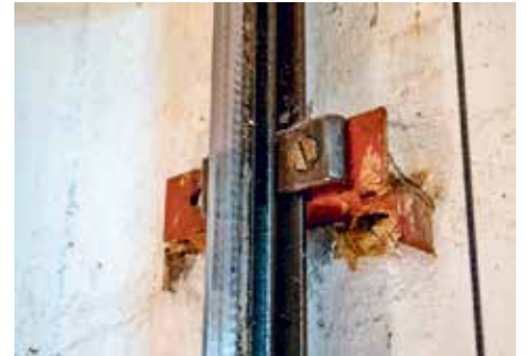
Old guide rails - here before renovation - have an almost unlimited service life.
