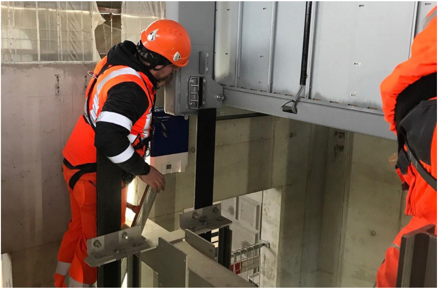
Lift installation in the south wing of Zurich main station.
